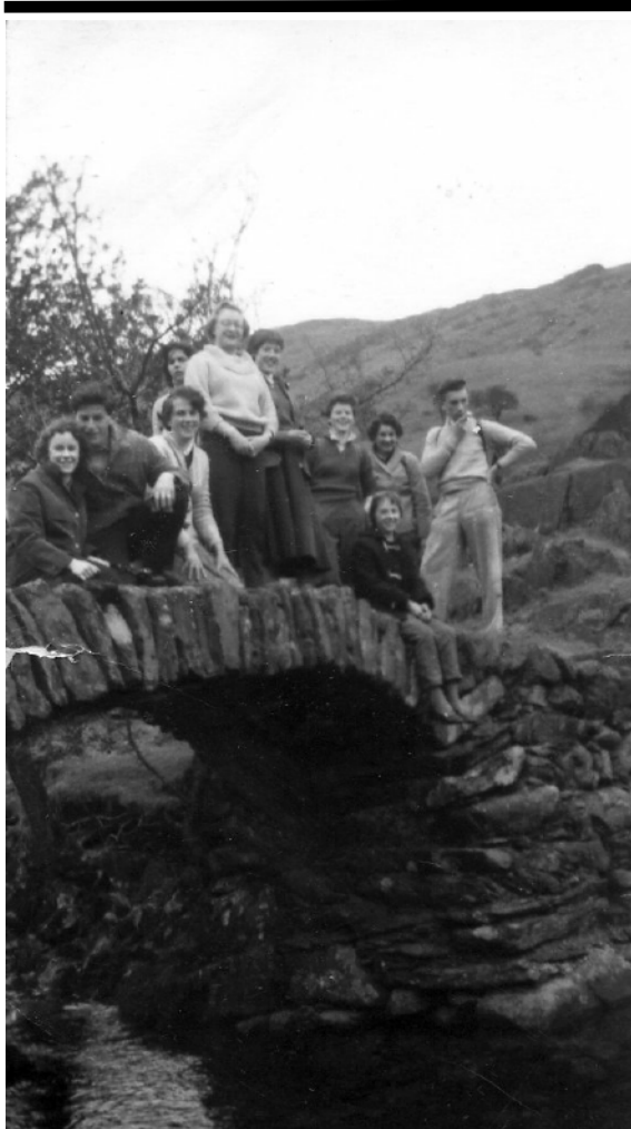
The rustic view above was taken on an Easter Lake District trip in 1957 and was sent in by MONICA JONES (53-59) now
